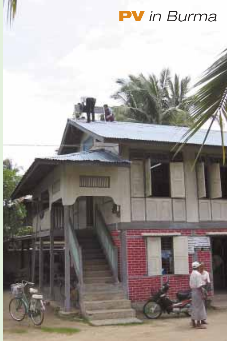
Above: Installing the panel on the Thaw Thi Kho Clinic roof.
