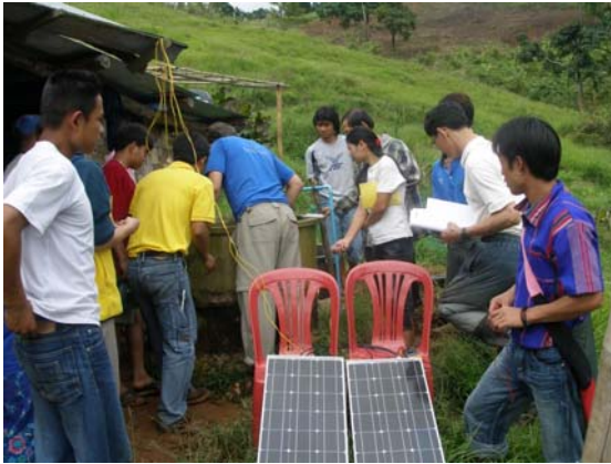
Solar pump installation.
