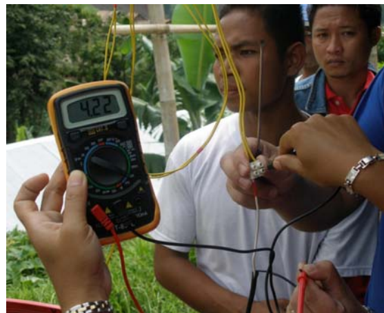
Measuring current output from solar panel.
