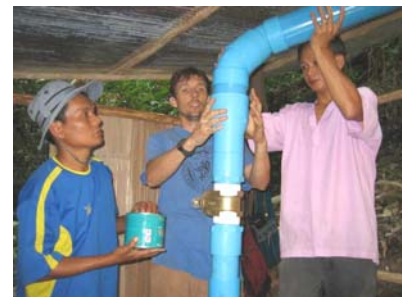
Penstock construction for micro-hydro Huai Kra Thing village, Tak Province.
