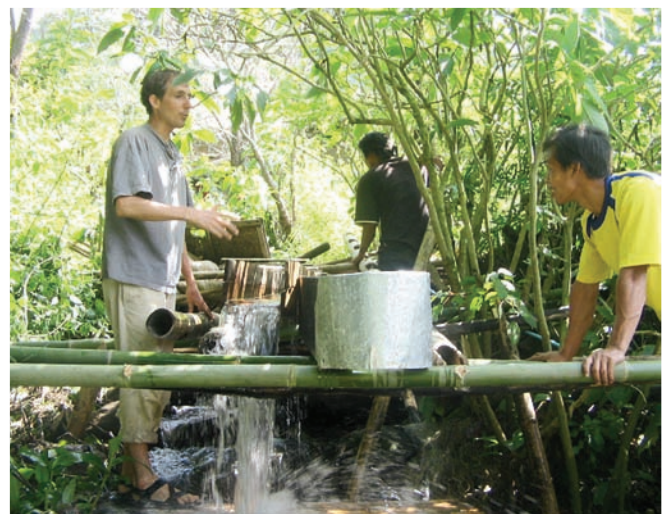
Chris and Somsak assemble the waterway.
