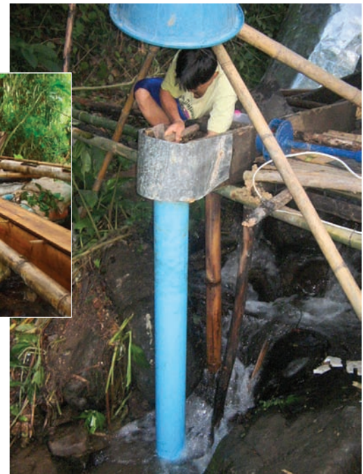
Above: The 6.5-foot-long draft tube is attached to the trough.
