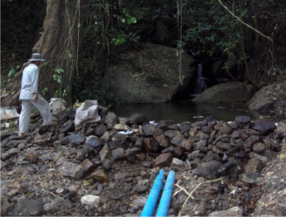
Figure 9: Completed dam. The dam is just high enough to ensure that the pipe inlets are submerged.
