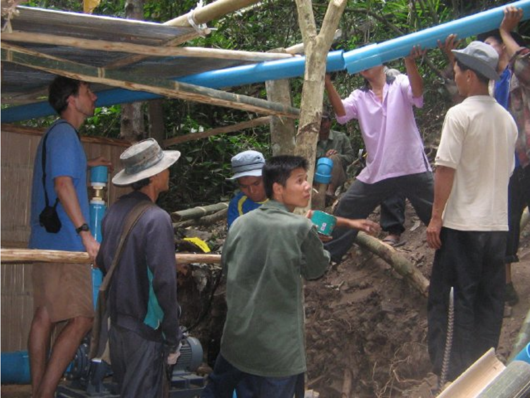
Figure 11: Connecting the penstock to the generator required careful alignment and some tricky angles.
