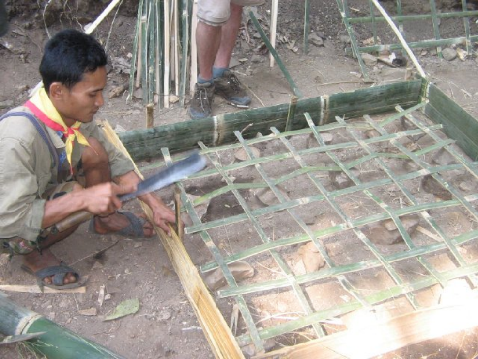
Figure 5. Surat sets bamboo form boards for cement pad that will hold the generator/turbine.
