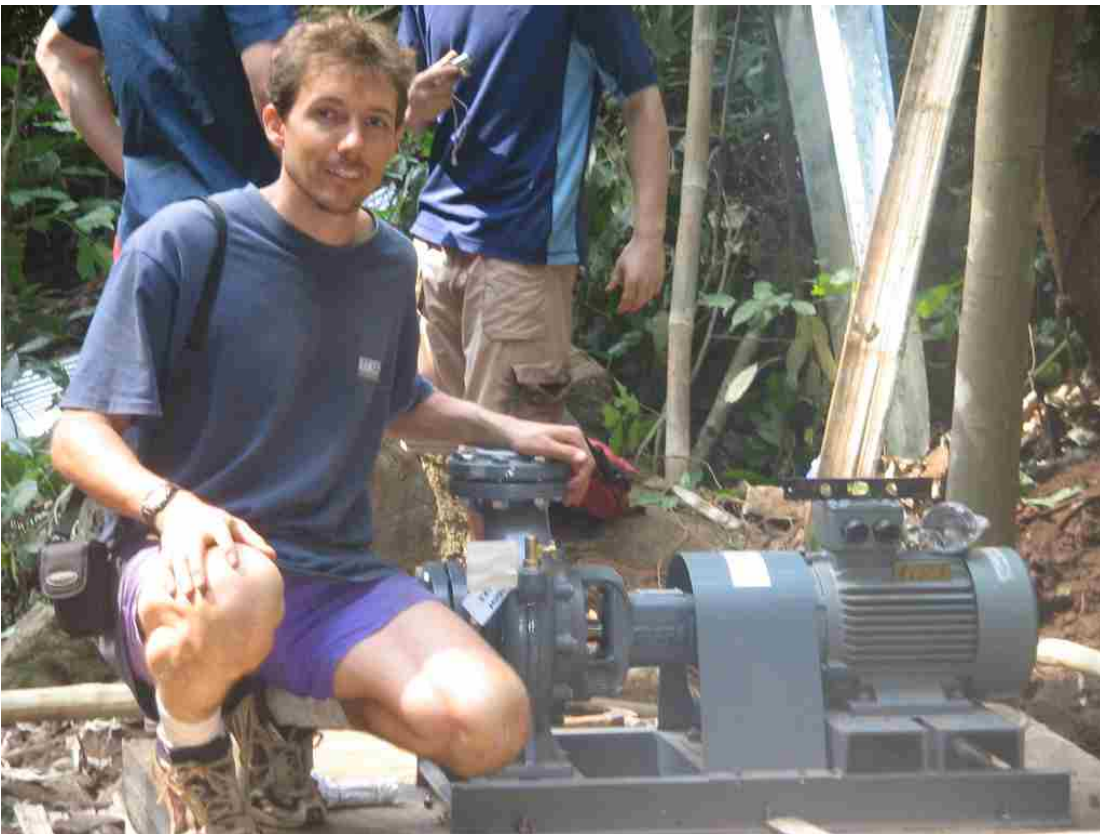
Figure 6: Chris poses by generator/turbine, now bolted to the cement pad. Chris' left hand rests on the pump outlet , which will serve as the inlet when operated as a turbine.
