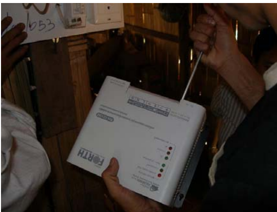
New Inverter Replacement
